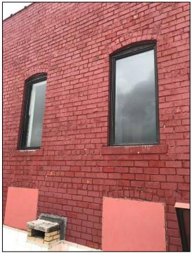
(3) We shall remove the existing polyurethane sealant from the window perimeters above the auditorium roof level. Upon completion, we shall install a new polyurethane sealant, tooled to a watertight condition. The color shall match the existing frame as closely as possible.
