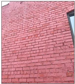
(1) All mortar joints above the roof level of the auditorium shall be cut back to a depth of two and one-half times the width of the mortar joints, but in no case shall the mortar joint be cut less than <sup>3</sup>/<sub>4</sub>-inch in depth. Once the cutting is completed, all surfaces shall be cleaned of all loose and foreign debris utilizing compressed air and/or pressurized water in preparation for repointing of the mortar joints.
